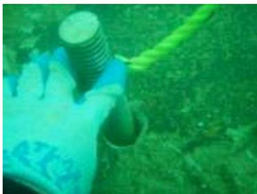
Q&S Engineering was contracted by Black & Veatch to install rock anchors into boulders at the toe of the causeway that were too large to be removed with a crane bucket. Q&S divers used air powered rock drills to install 1 ¾ stainless steel Williams Rock
